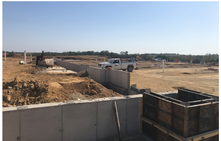
Area B and C Foundation Walls
