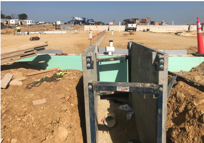
Area B & C Underground Plumbing
