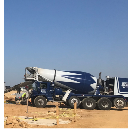
Concrete Mixer Truck Delivering Concrete for Area B Foundation Walls
