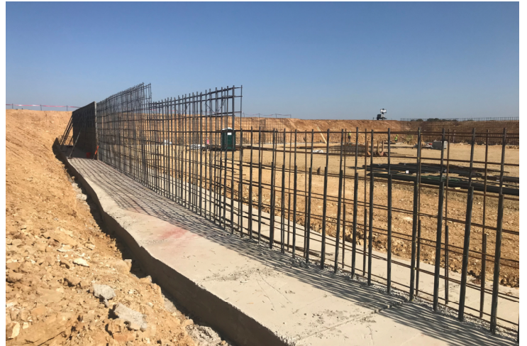
Rebar Tying for Gym Retaining Walls
